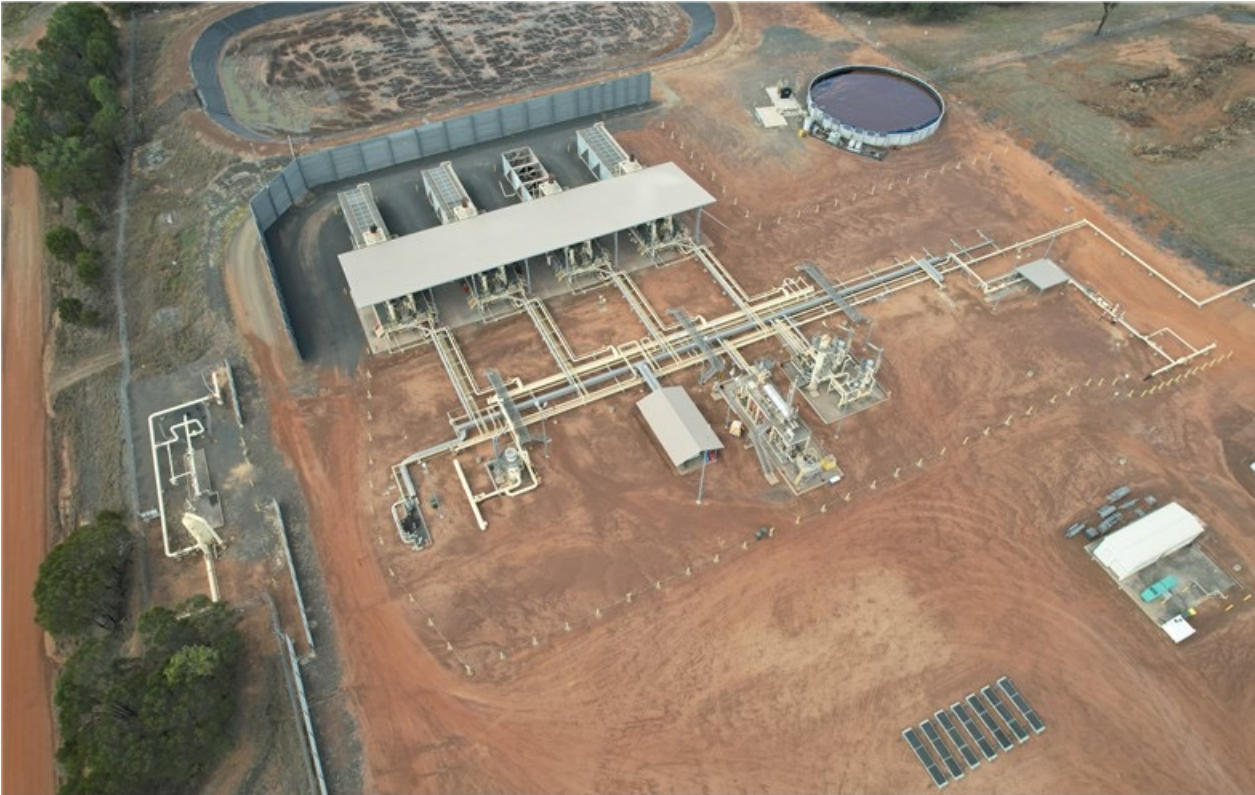
Moranbah Gas Processing Facility
